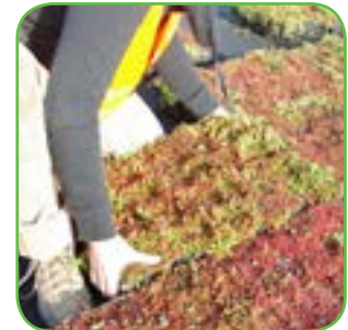
Hooking HYDROPACK® trays
