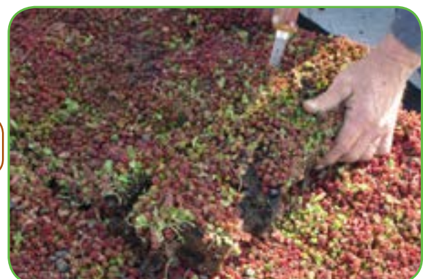
Cutting the vegetation and soil with a knife, keep the filter
