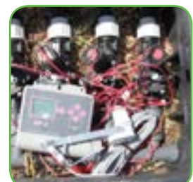
Irrigation electro valves
