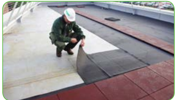
Inspection of the membrane and the protection fabric
