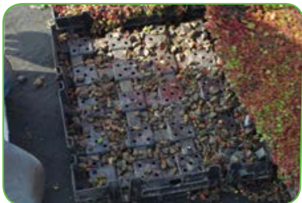
Placing the mineral drainage back into the reservoirs
