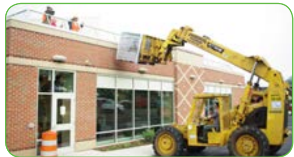
Lifting the HYDROPACK® pallet onto the roof
