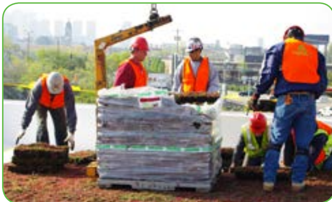
HYDROPACK® pallet lifted by crane
