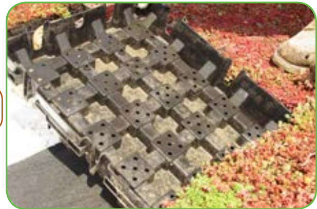
Placing the tray with edges facing outward
