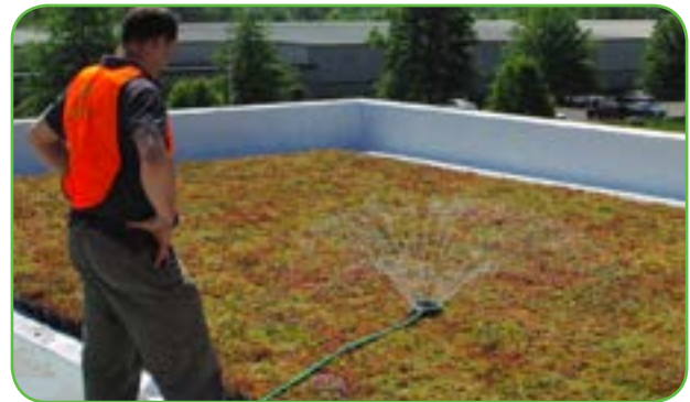
Watering after installation – this small sprinkler must be repositioned to ensure that the entire roof receives the correct amount of water.
