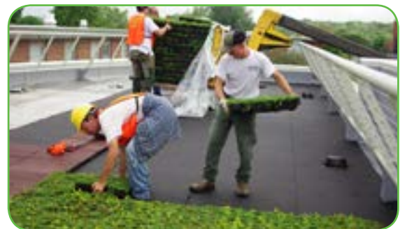
HYDROPACK® installation
