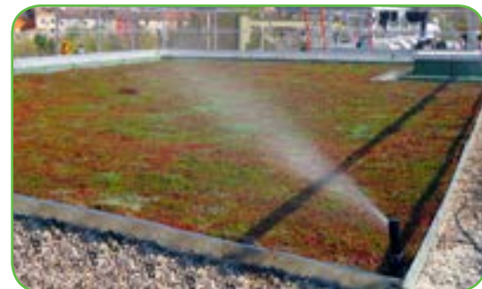
Permanent overhead irrigation
