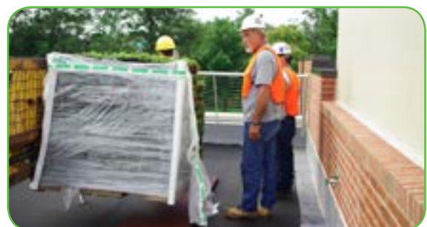
HYDROPACK® pallet on the roof
