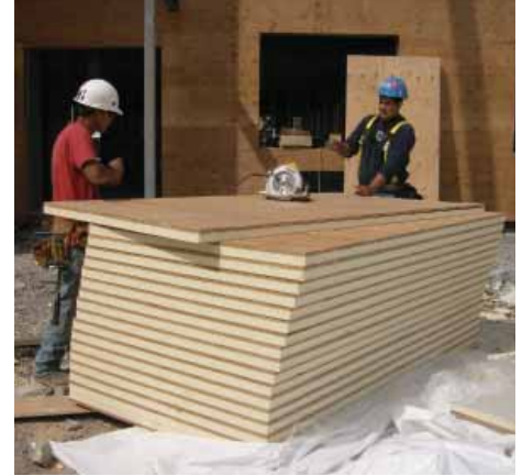
R2+ BASE 4' x 8' boards, installed directly over steel studs
