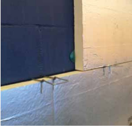
R2+ SILVER, 16" X 8' boards installed between rows of embedded brick ties
