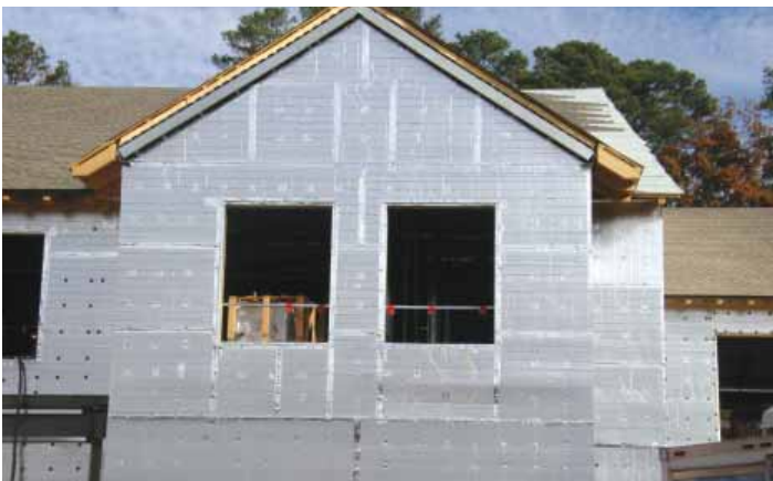
R2+ SHEATHE 4' x 8' boards fastened directly over studs, joints taped with CCW Foil-Grip 1402
