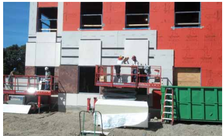
R2+ MATTE 4' x 8' boards installed over exterior gypsum sheathing and WRB
