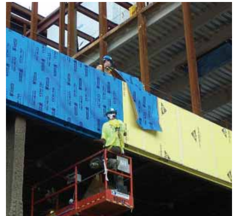
CCW-705 installation over Exterior Gypsum Sheathing
