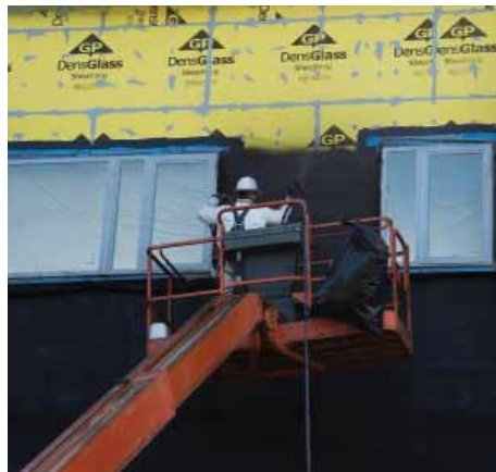
Barriseal-S with CCW-705 Flashing & Polyurethane Caulk Details
