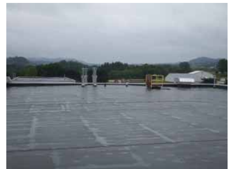
Polyiso Insulation can handle high temp and humidity, directly beneath a black membrane
