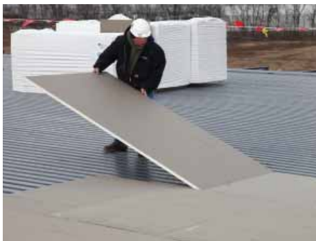
Polyiso Insulation being Installed on a Roof Deck
