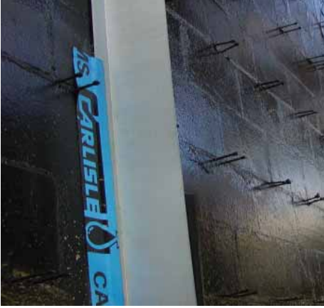
Barriseal-S on Concrete Block Wall with Embedded Ties
