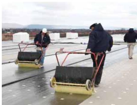
Polyiso Insulation Accepting Bonding Adhesive and a Roof Membrane
